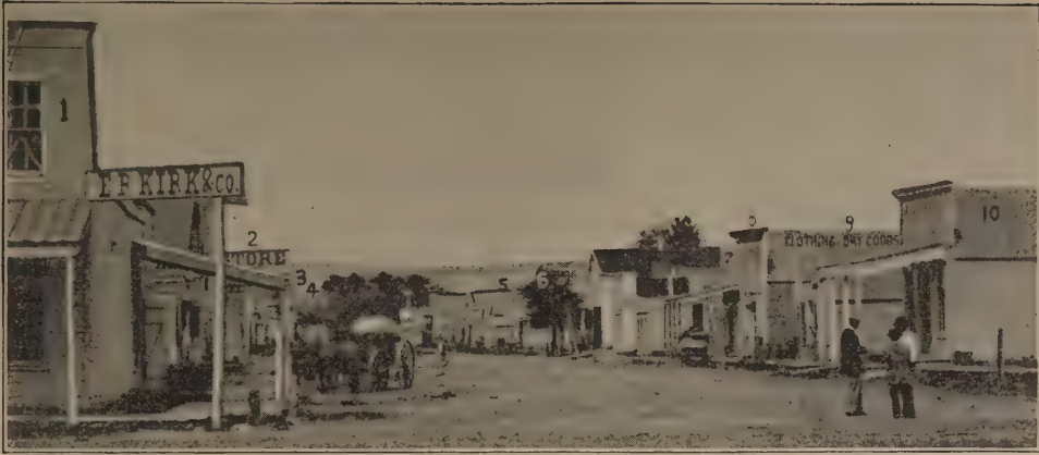
SIoux CITY, LOOKING NORTH ON PEARL STREET FROM SECOND STREET, AUGUST, 1866
